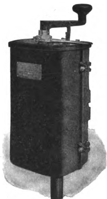
Fig. 1778—Master Controller for Type H. L. Control, Closed
