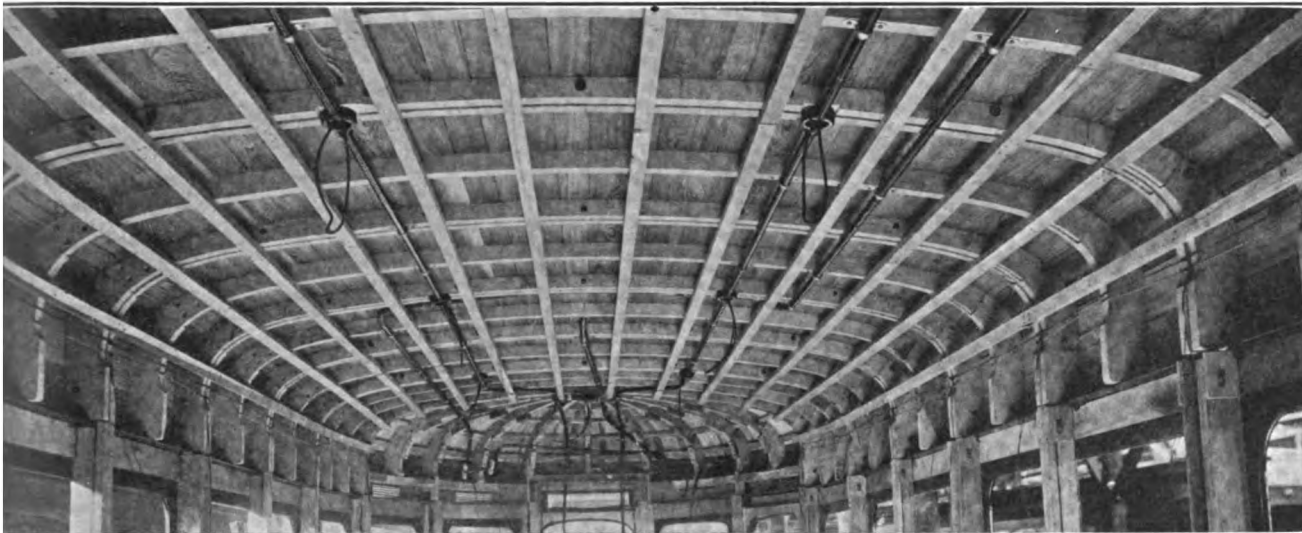
Fig. 1845—Metal Conduit in Roof Framing with Condulet Outlets for Deck Lamps
