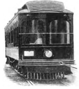
"Heavy Weight" Anti-Climber for Interurban Cars 5½" x 2" Rolled Steel
