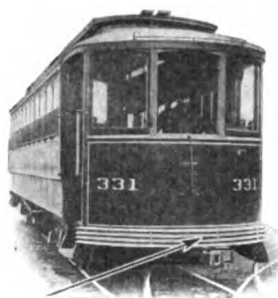
"Light Weight" Anti-Climber for City Cars 7" x 1" Rolled Steel
